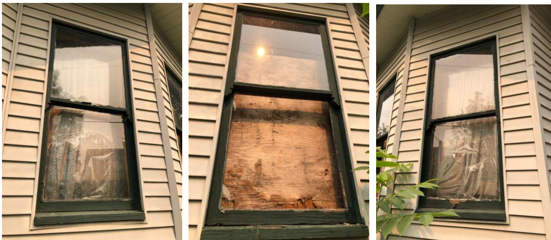
Figure 17b: Bay windows, south side (left, centre, right)
