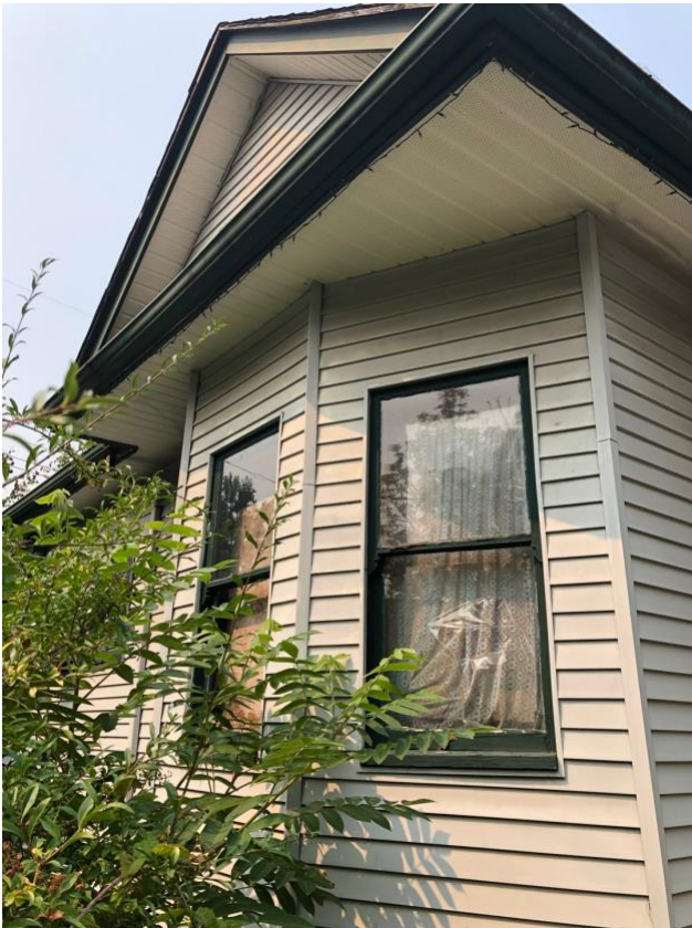
South side bay window and gabled roof extension above.
