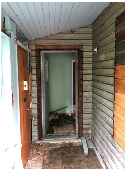
Figure 15: Original front door opening from the porch (centre); added front door on outer face of porch (left).
