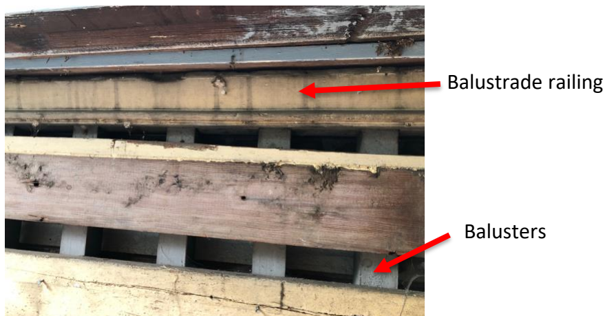
Figure 12: Balustrade with balusters visible behind horizontal enclosure boards
