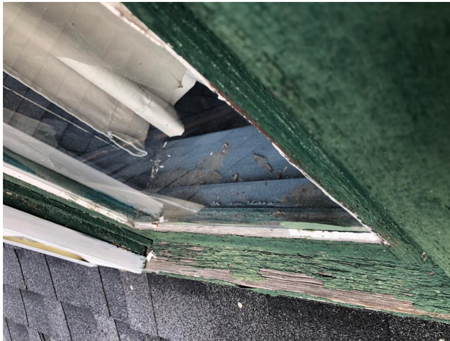
Figure 18a: Attic dormer window, sill and trim – west side (front).
