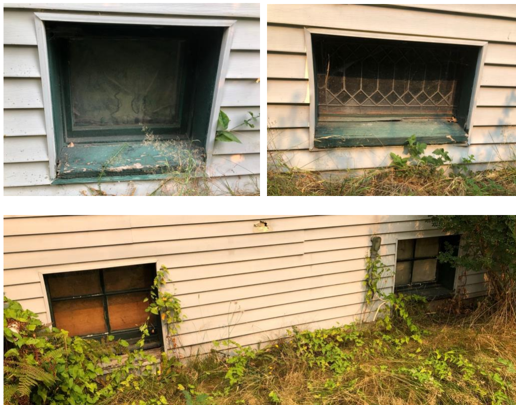
Figure 16: Basement windows, south side – clockwise from top: below porch, below front room, below kitchen.
