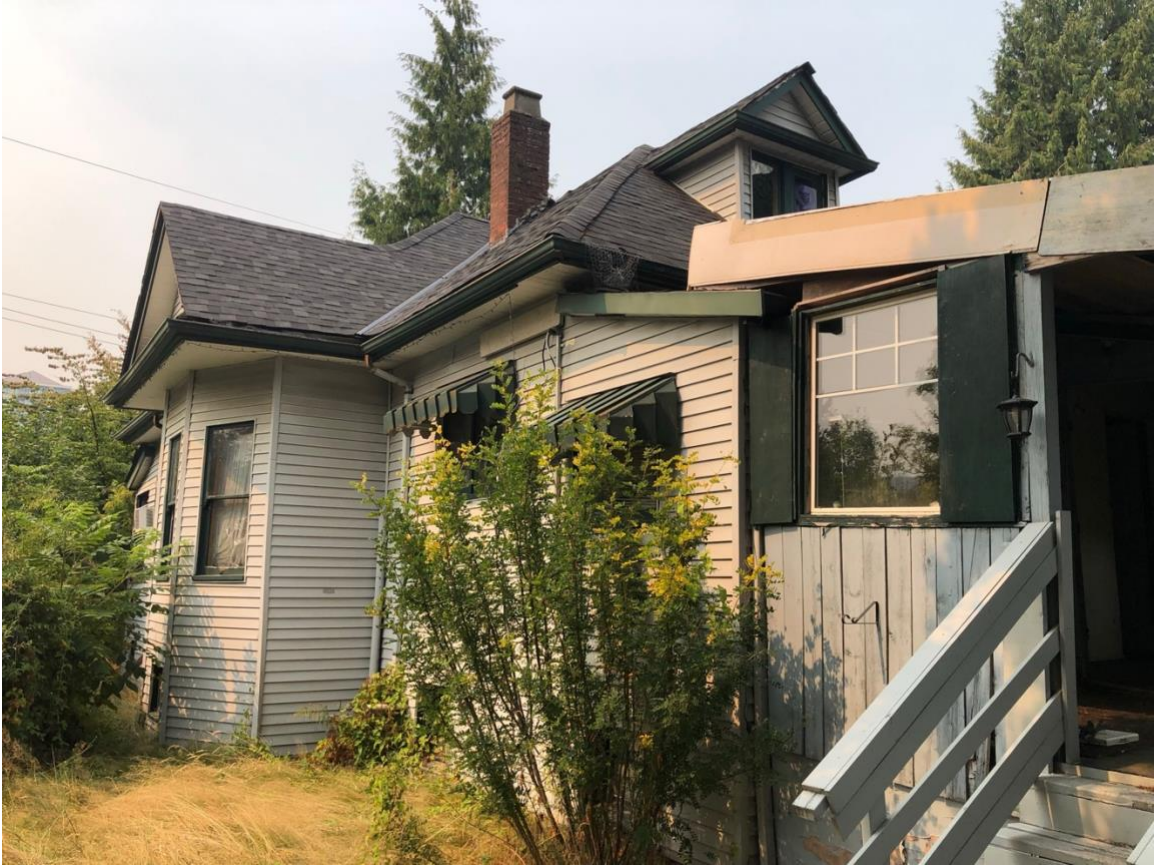
South side and rear shed roof extension, with covered rear porch.
