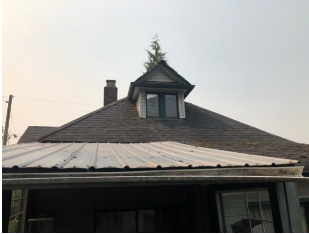
Figure 19b: Roofing as seen from the rear
