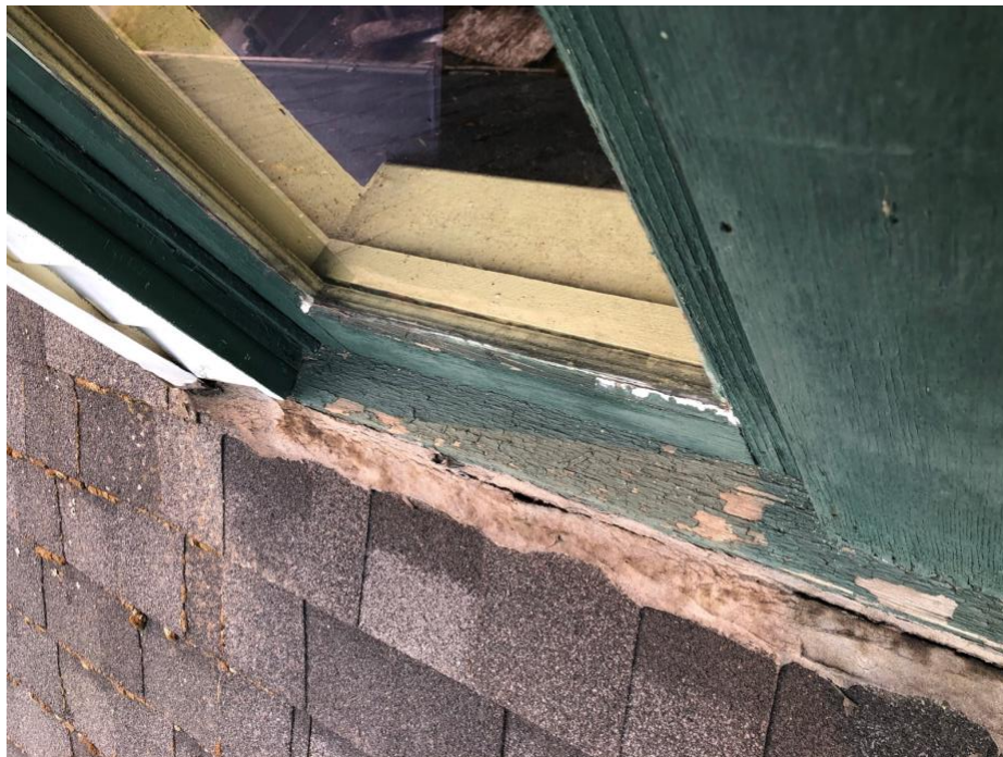
Figure 18b: Attic dormer window, sill and trim – east side (rear).
